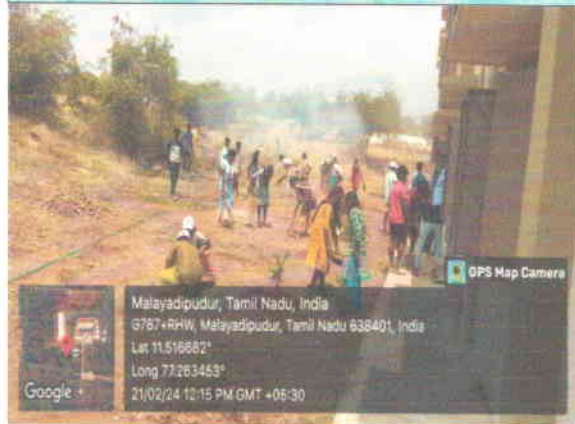
CLEANING NEAR KAMARAJAR BLOCK
